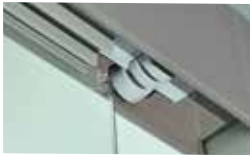
2 Sensor technology to detect the sash position
