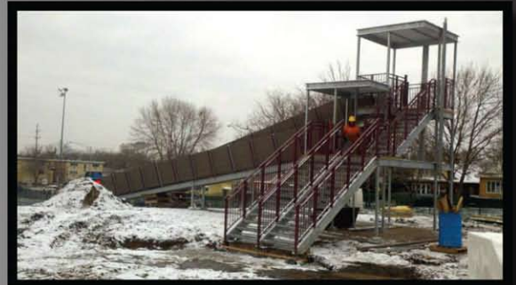
Blue Island Launch Structure Blue Island, IL
