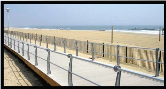
Boardwalk Posts and Handrails Spring Lake, NJ
