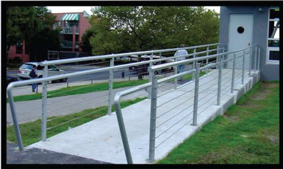
Pedestrian Railings Starlet City, Brooklyn
