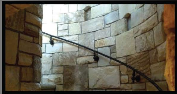
Residential Construction Stairwell Vestal, NY
